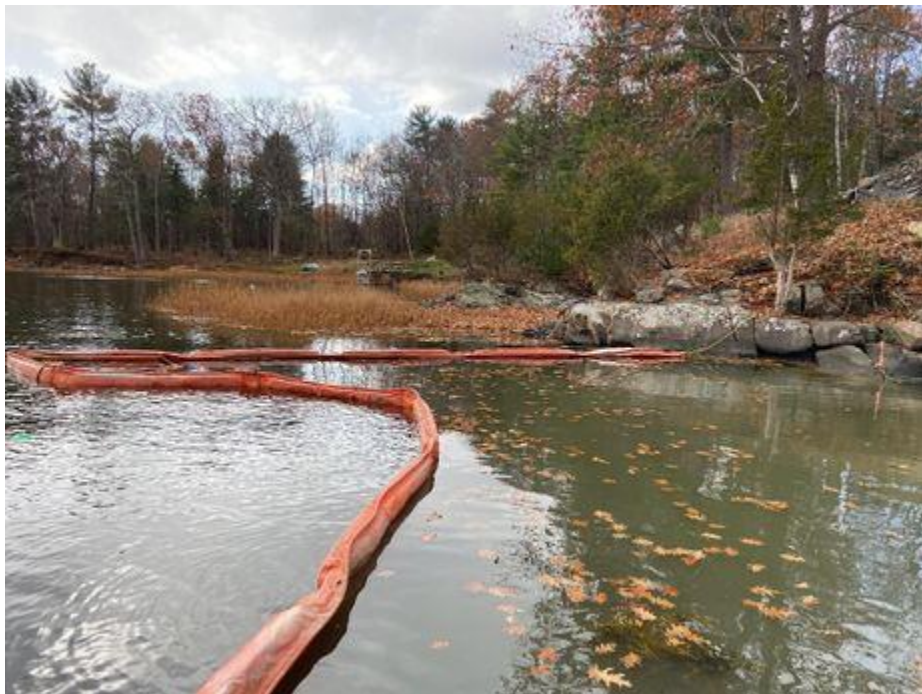
Photo 4. Turbidity barrier, view south, Durham, NH.
