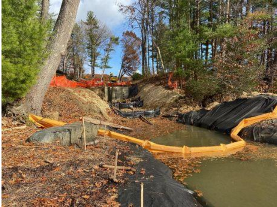
Photo 6. Cable trench, view east, Newington, NH.
