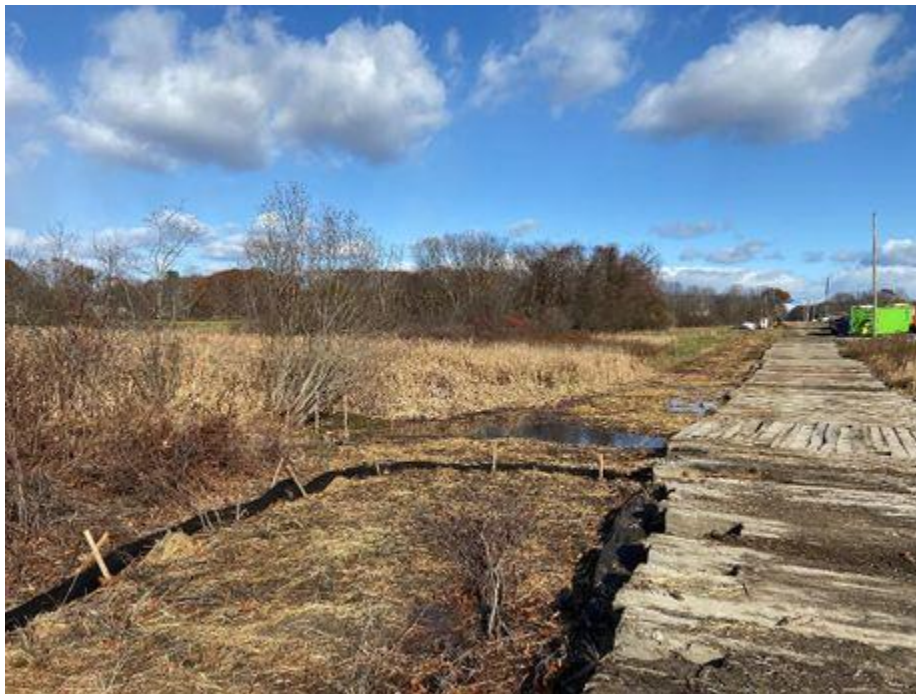
Photo 10. Wetland NW16 erosion controls, view east, Newington, NH.
