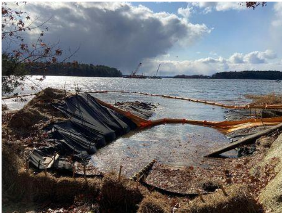
Photo 8. Turbidity barrier, view southwest, Newington, NH.
