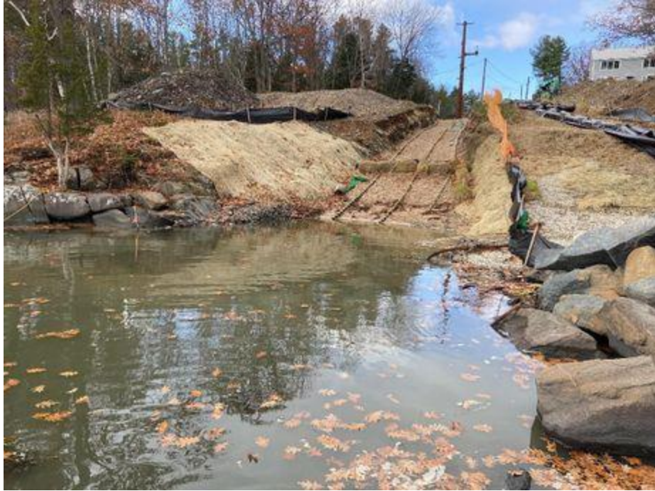
Photo 3. Cable trench, view west, Durham NH.
