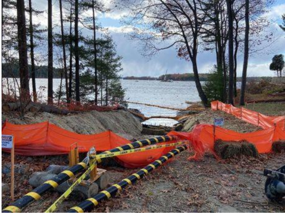
Photo 5. Cable trench, view southwest, Newington, NH.
